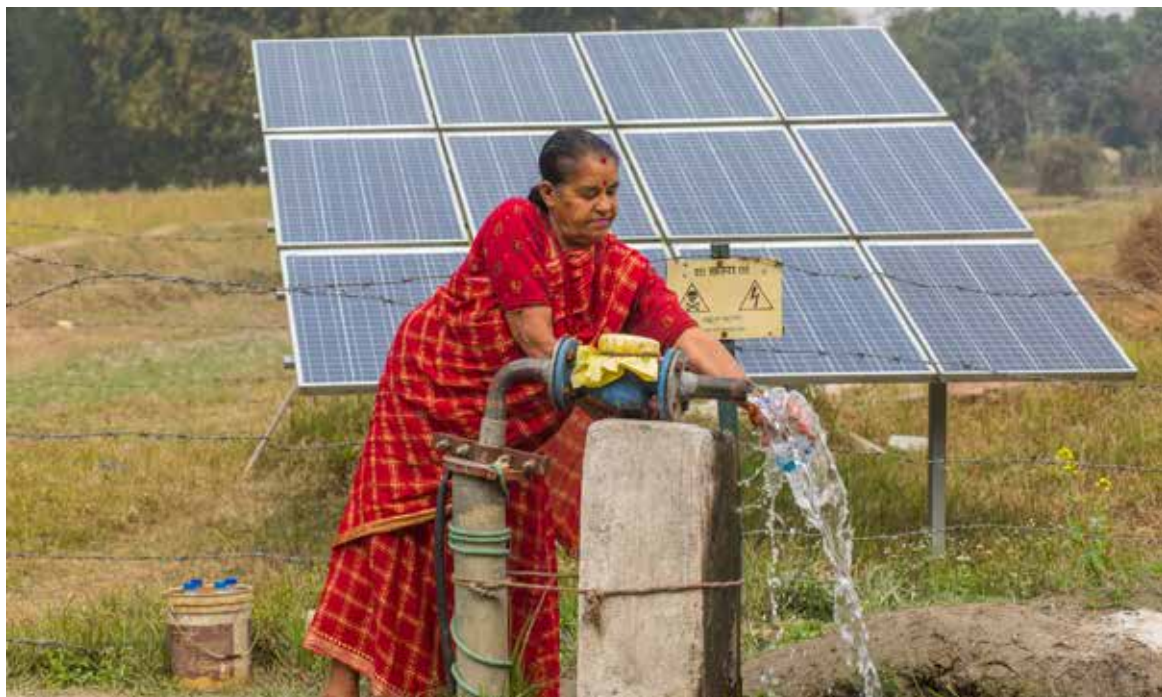
A farmer with her solar irrigation pump in Saptari District of Nepal.© Nabin Baral/IWMI via Flickr
