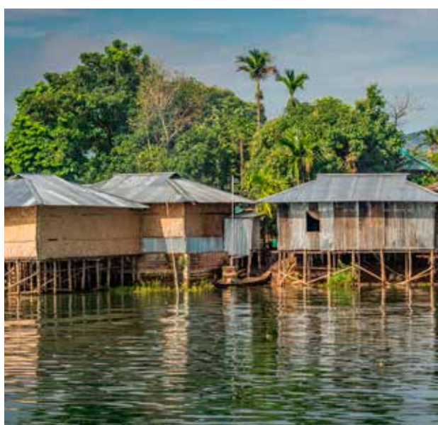
A row of stilt houses in Bangladesh to help face the yearly devastation from the floods. © StevenK via Shutterstock
